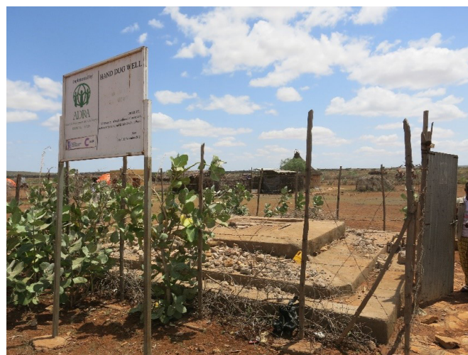
Broken water pump in Somali
