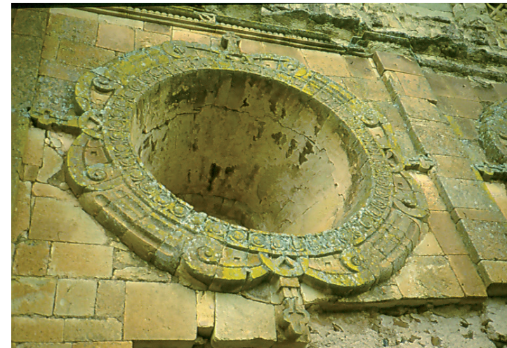
Window in one of the walls of the church of Gorgora
