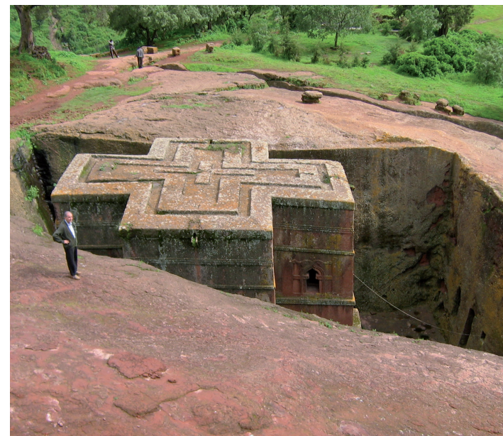
Roof of the church of St George
