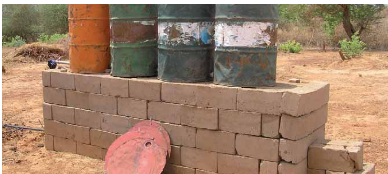
Photo 10. Reservoir. Ville de Kayes, Kayes.
