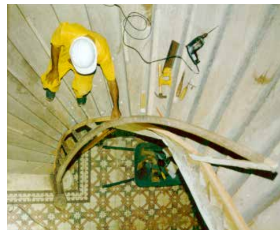
▲ Balustrade restored. Carpentry workshop ▼ Plastering and painting workshop
