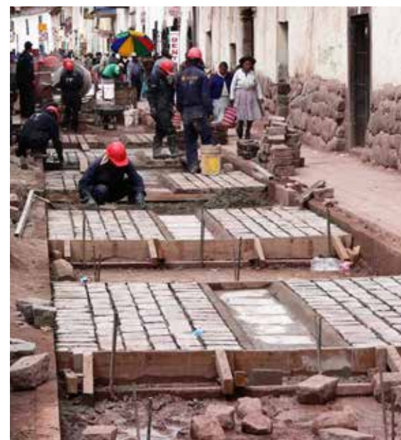
▲ Calle Hospital. Bricklaying and stonemasonry workshop ◀ Carpentry workshop
