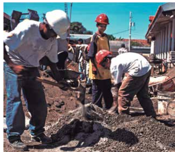
▲ Former Comando building. Construction workshop ◀ Metalwork shop
