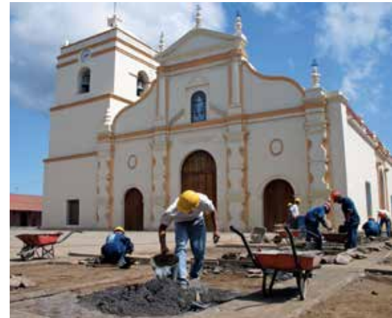
▲ La Asunción Parish Church. Construction workshop ◀ Electricity workshop
