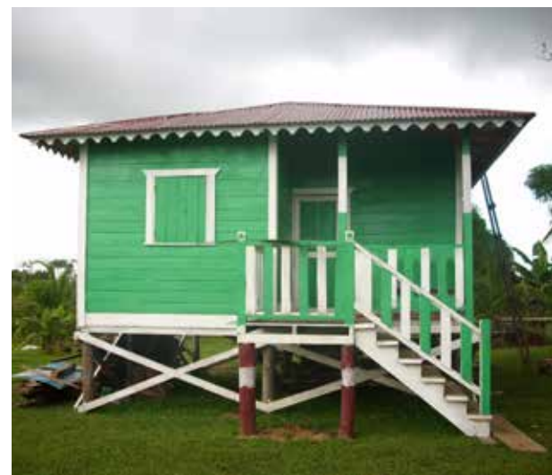
House built in Tuara: In progress Finished product
