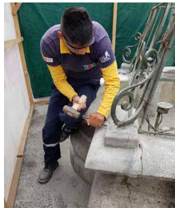
▲ Plaza San Lázaro. Bricklaying/stonemasonry workshop ◀ Quinta de Presa. Carpentry workshop
