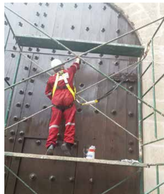
▲ Church of St Francis. Carpentry workshop ▼ Ransom Room. Maintenance work
