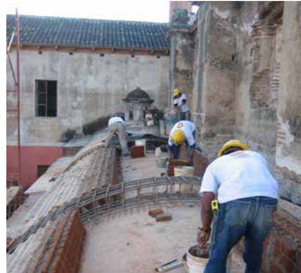
▲ Company of Jesus. Construction north dome ◀ Antigua villages. Park maintenance
