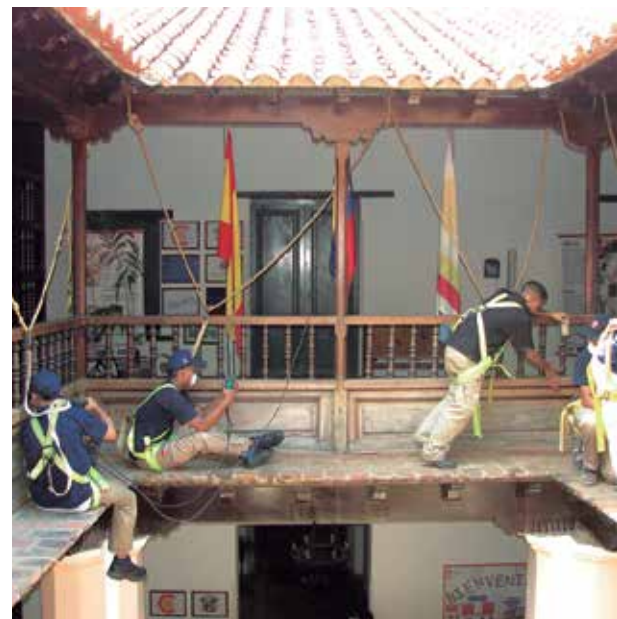
▲ Casa Boulton. Carpentry workshop ▼ Metalwork shop
