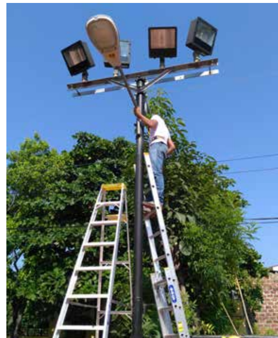
▲ Electricity workshop ▼ Hato Hasbún Sports Centre. Construction workshop
