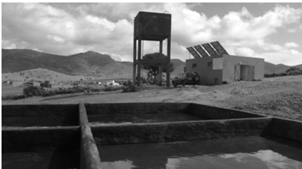
FIGURE 4. PV-RO SYSTEM INSTALLED IN TANGARFA (MORROCCO) (SOURCE: ITC).
