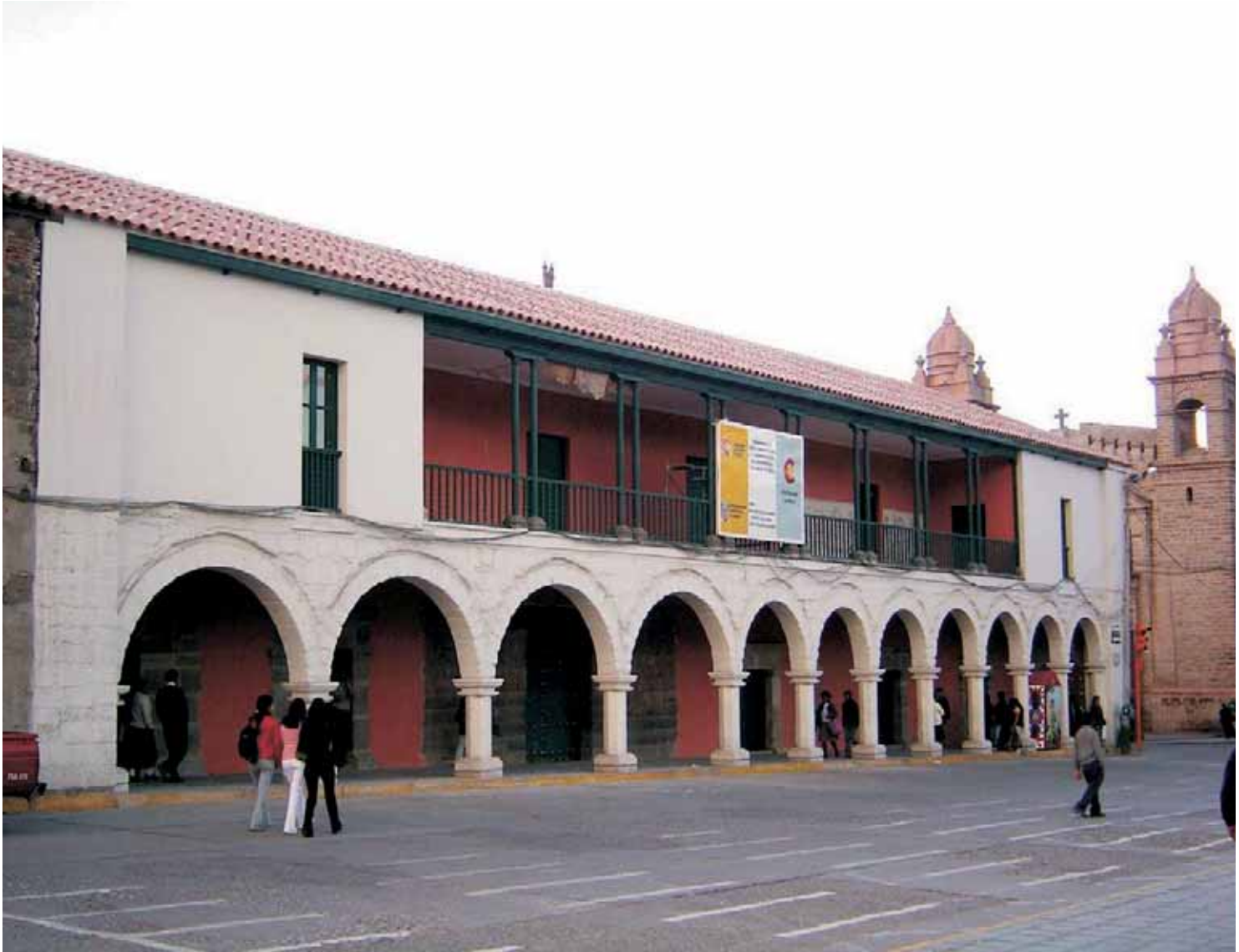
Fachada principal restaurada
