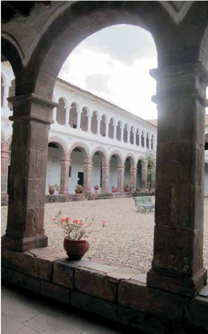
Claustro principal restaurado
