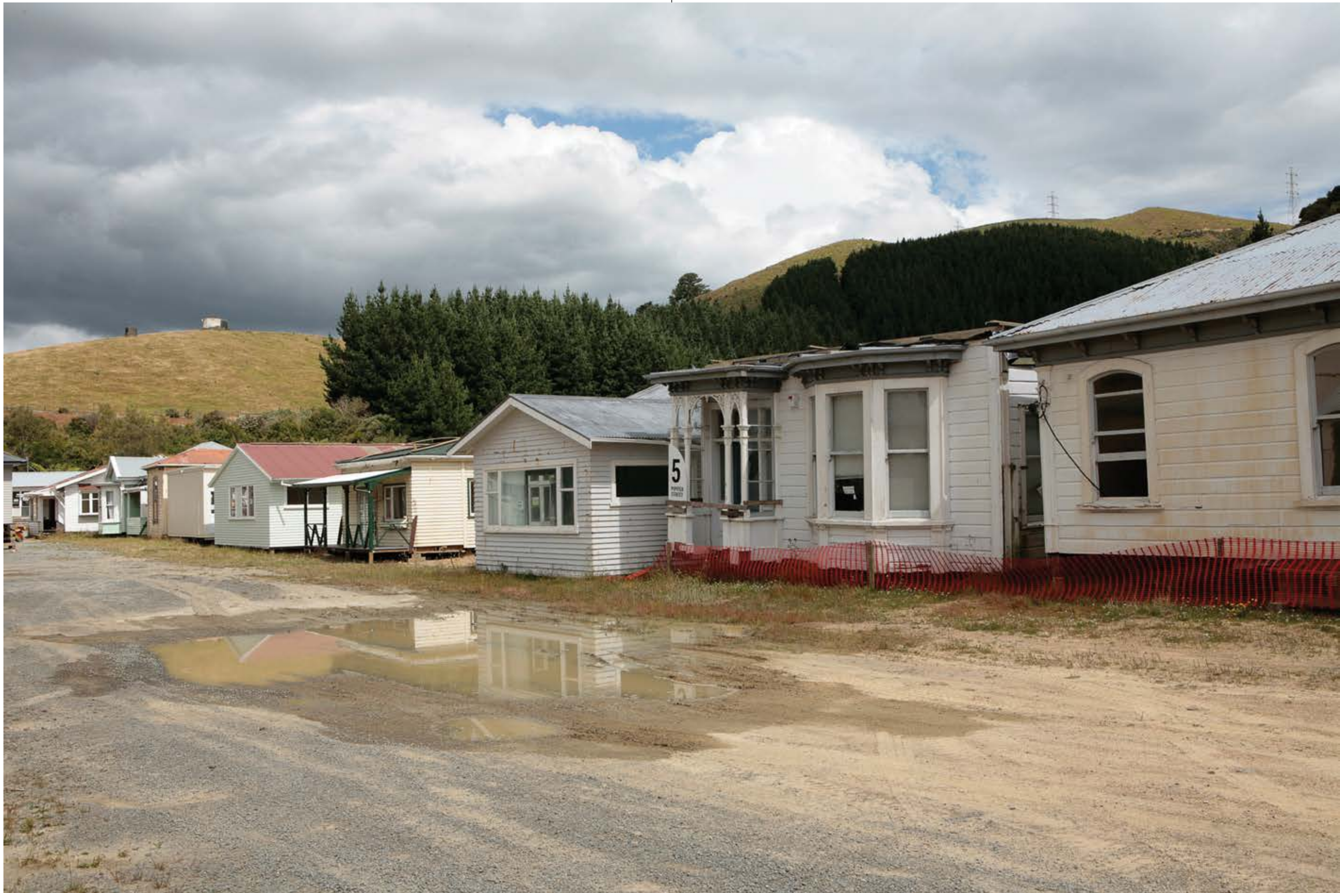
Casas reubicadas / Relocated houses / Britton's Yard, Wellington, 2009
