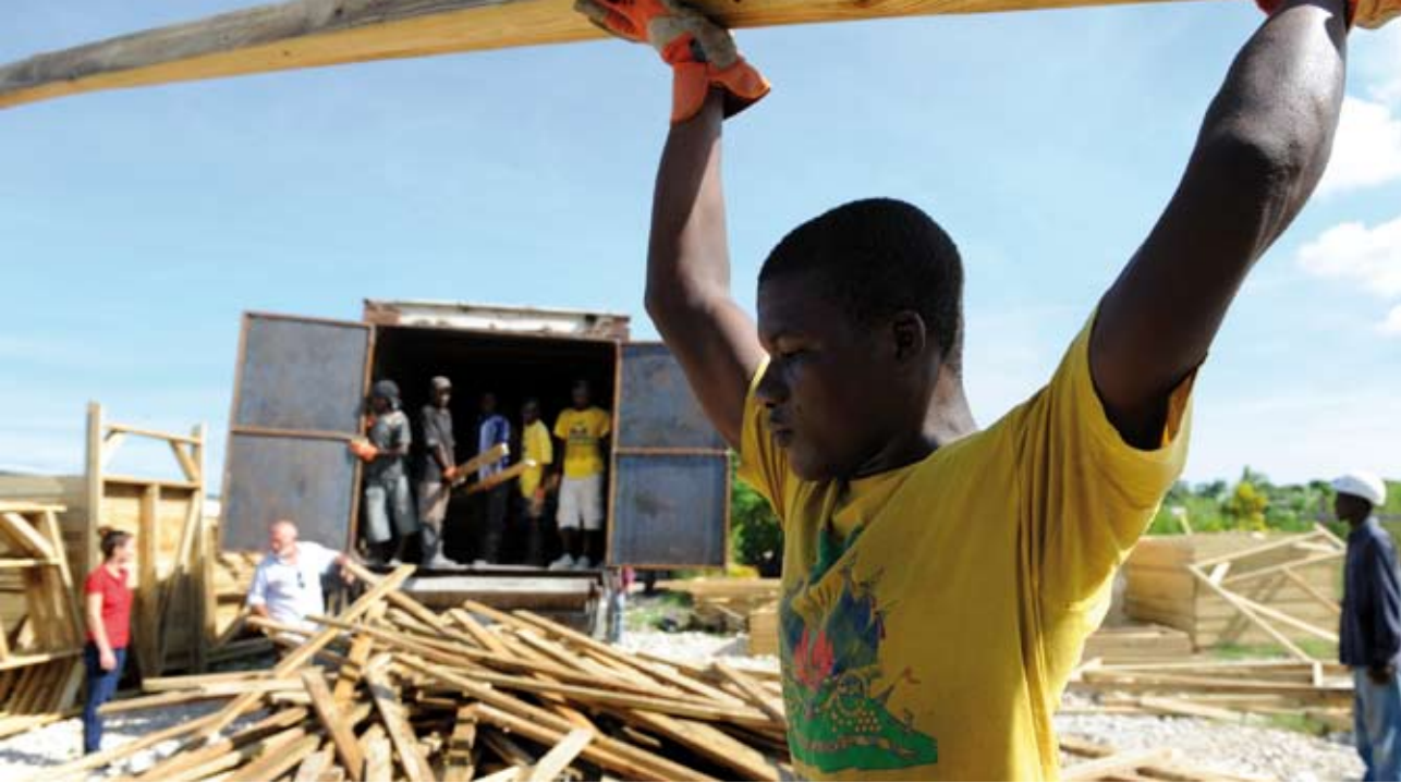
Workers prepare materials for temporary shelters. Source: USAID/Kendra Helmer
